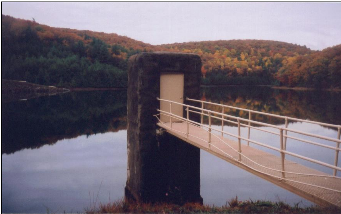
Figure 5: Exterior of Intake Tower Structure above Reservoir Level
