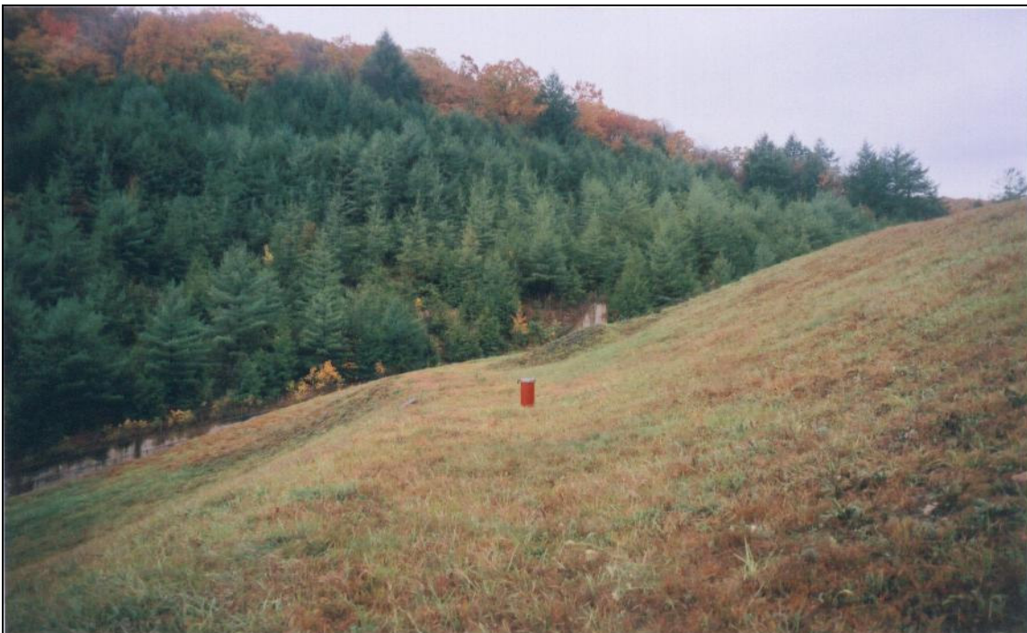
Figure 2: Piezometer Along Bench #1
