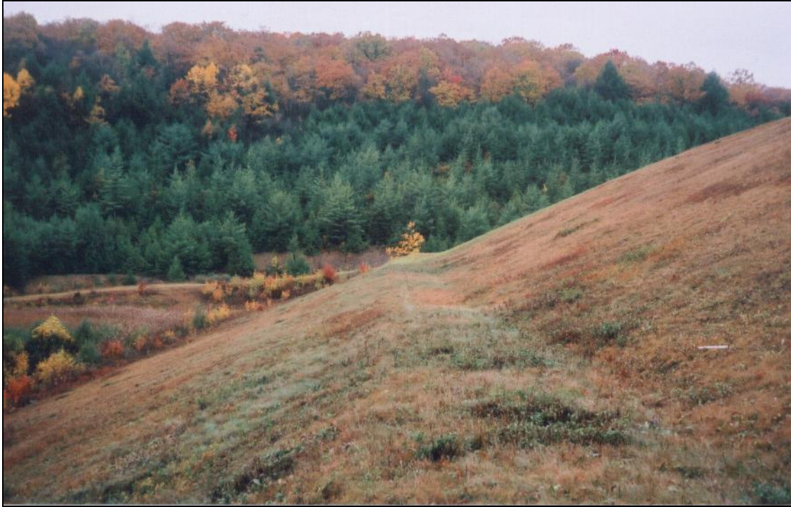
Figure 1: Bench #2 Added for Embankment Stability
