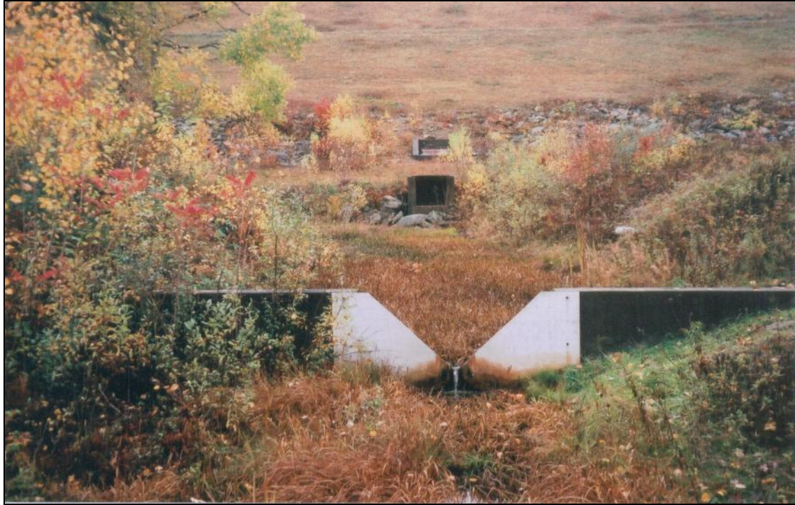
Figure 4: V-Notch - Seepage Monitoring Weir
