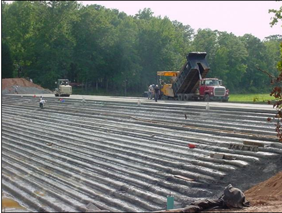
Figure 9: Typical RCC Construction (Courtesy of www.agpeltz.com )
