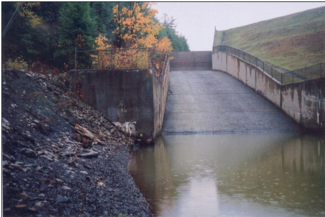
Figure 7: Spillway Discharge Basin
