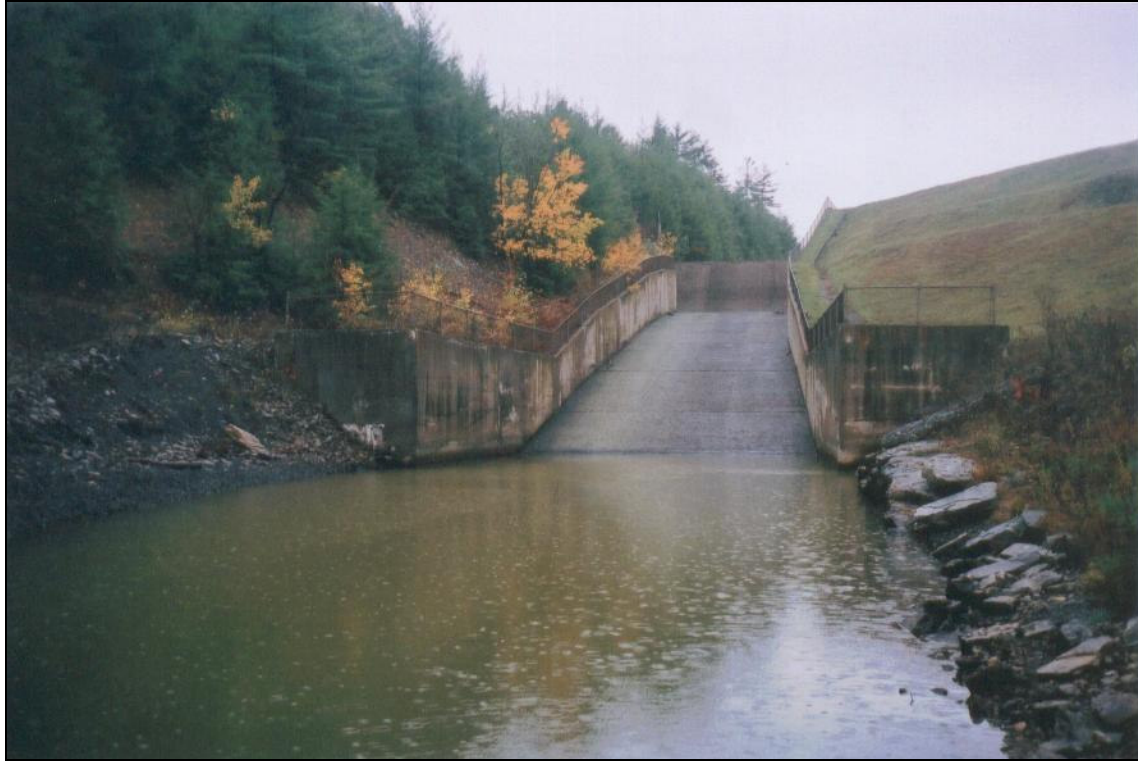
Figure 6: Spillway Chute, Looking Upstream
