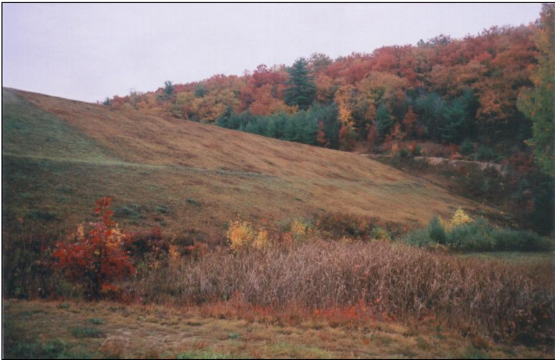
Figure 3: Overall Downstream View of Dam
