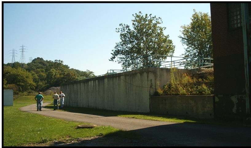
Side View of Sedimentation Basin
