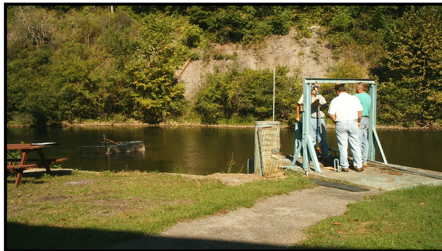
Intake Chamber (On Right)
