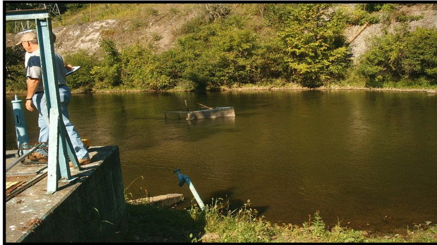
Diversion Structure at Raw Water Intake
