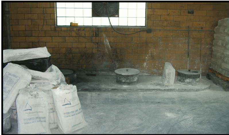
Dry Chemical Hopper Loading Area
