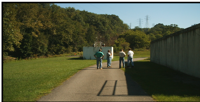
Wastewater Holding Tank (Background)
