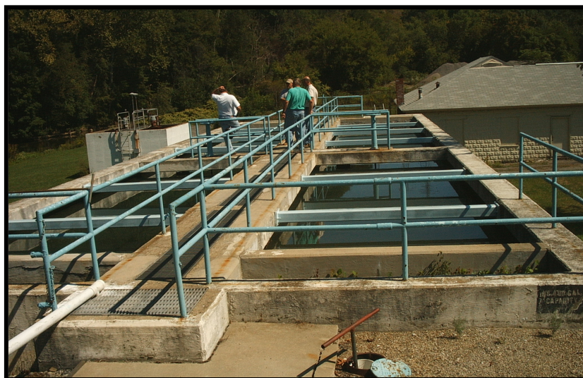
Top of Sedimentation Basin
