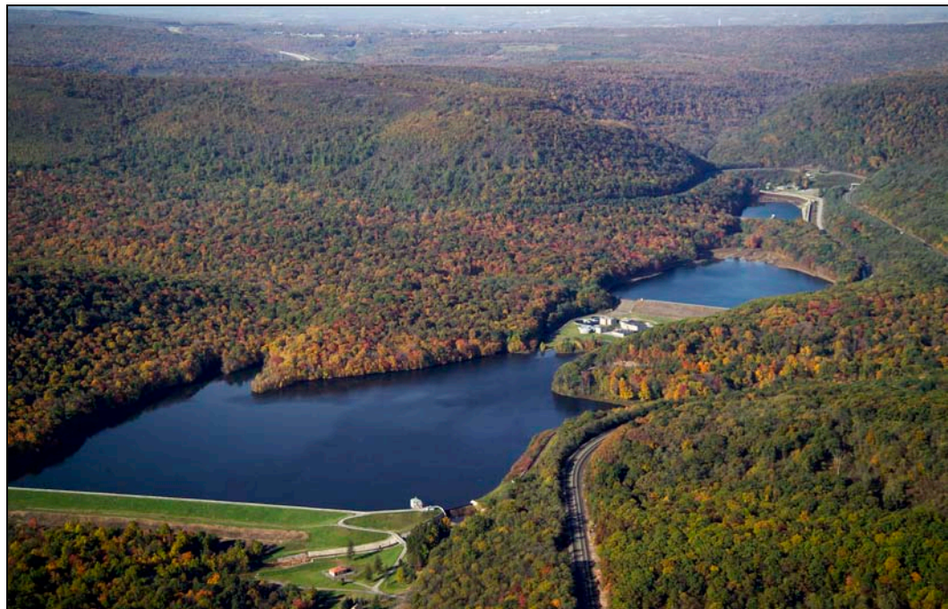
Photo No. 11 - Horseshoe Curve Reservoir Systems
